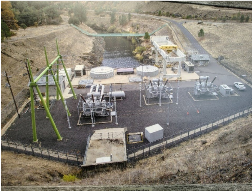
Figure 4.9.1.1-7: Collierville Powerhouse and Tailrace
